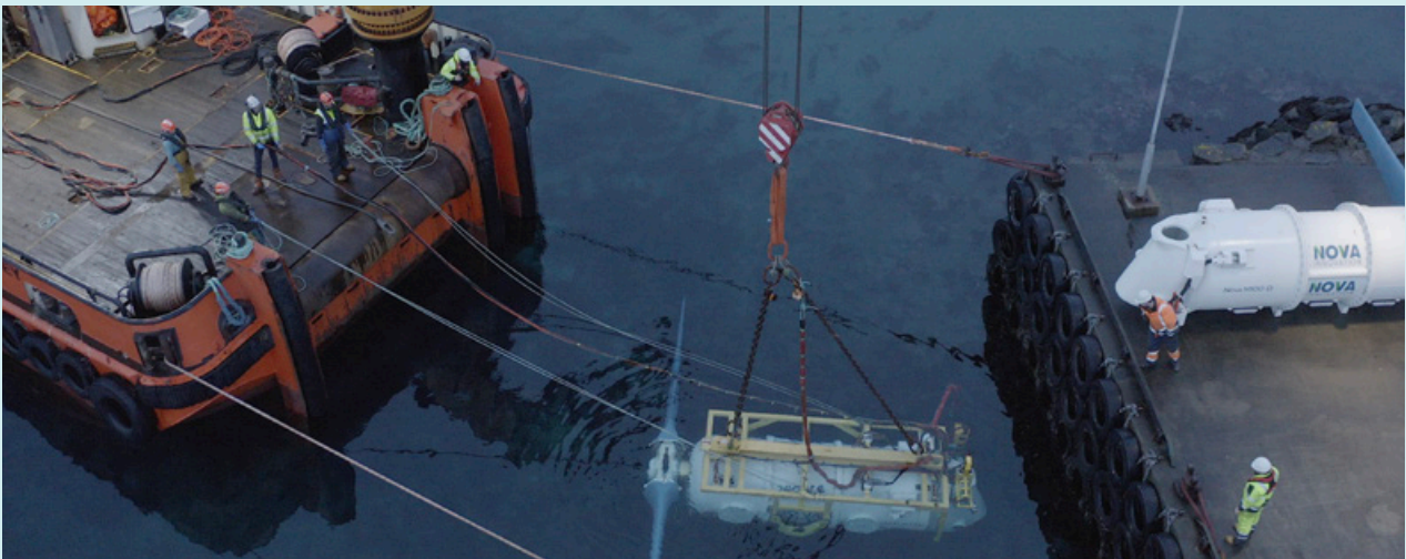
Deployment of turbine 5, Grace, for Nova Innovation (Credit: Nova Innovation)
